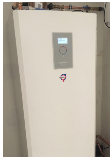
Thermia Comfort Optimum,, grond-bron warmtepomp
